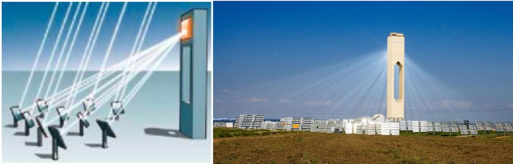
**Fig 1. Left: a schematic representation of central receiver technology.. Right: the Abengoa PS10 power tower in operation near Seville, Spain.**
